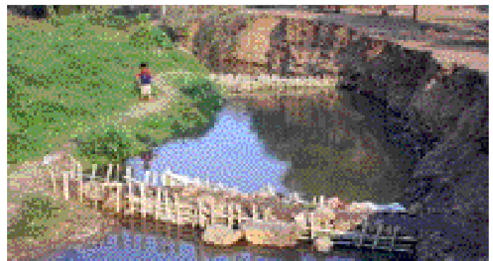
Check dam in operation
